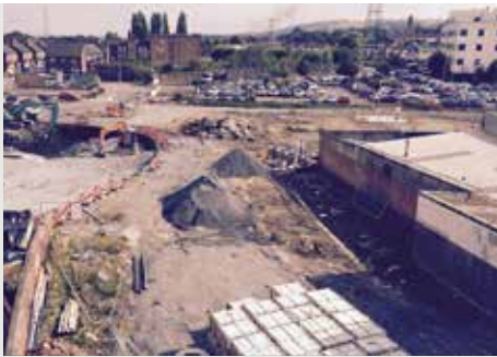
C.S. Lewis Square Under Construction
