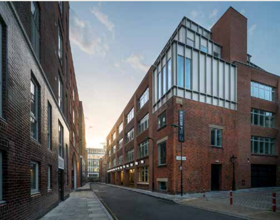
Below: Example of new commercial accommodation built on top of existing building
